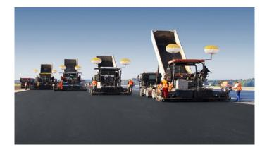
Having a detailed 3D model of the existing surface in advance of works commencing allows successful planning for accurate material calculations and eliminating guesswork for quantities of asphalt or milling required. SmoothRide is the perfect tool for mainline paving or milling projects requiring long sections of road that need resurfacing. This complete workflow allows you to stay productive and be ahead of schedule.
